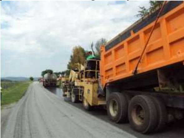
Oil is sprayed on the road surface by an oil tanker, followed by a chip machine that tows a dump truck while spreading stone on the oil. The operation is completed when a roller permanently embeds the stone in the oil.
