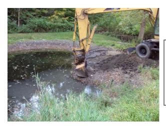
We cleaned out accumulated debris from the pond on Center Hill Road for the Fire Co. These ponds with dry hydrants are important to the fire company to maintain public safety. The hydrant in this pond was unusable until we dugout the material covering the intake pipe.
